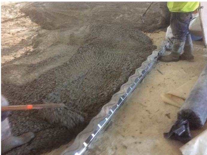
Pouring the first side.
