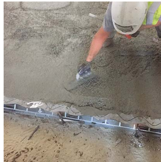
Finishing with a hand trowel.
