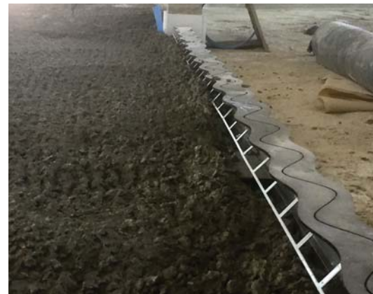
Continuous concrete ties ensure firm anchoring into the slab.
