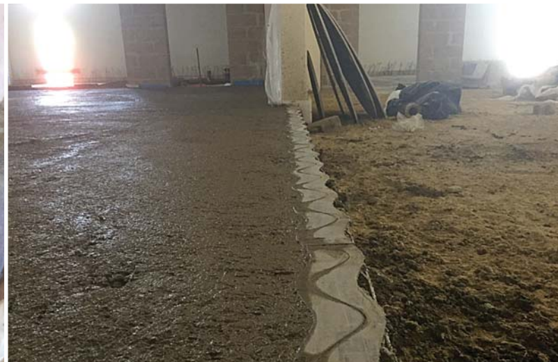
The first side, ready for power trowelling.
